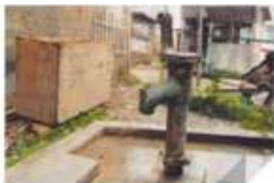
Figure 46. Deserted hand tubewells either fail to extract groundwater or yield arsenic-contaminated water. Source: Photo credit: Samad, 2003, personal communication
